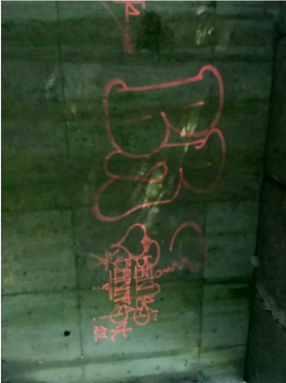
Right Bank Abutment when facing downstream
